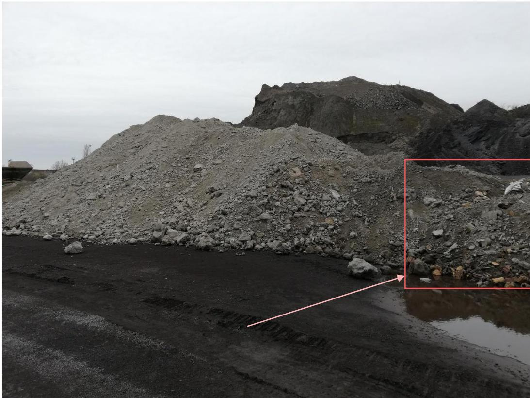
*Figure 20: Starting stockpile ( arrow indicating the part of slag with too many exogenous elements removed directly)*
