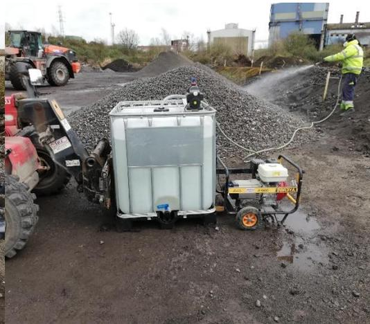
*Figure 26: Spraying acetic acid solution*
