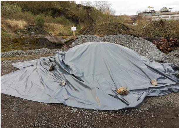
*Figure 25: Crushed 0-10 put under a tarpaulin*
