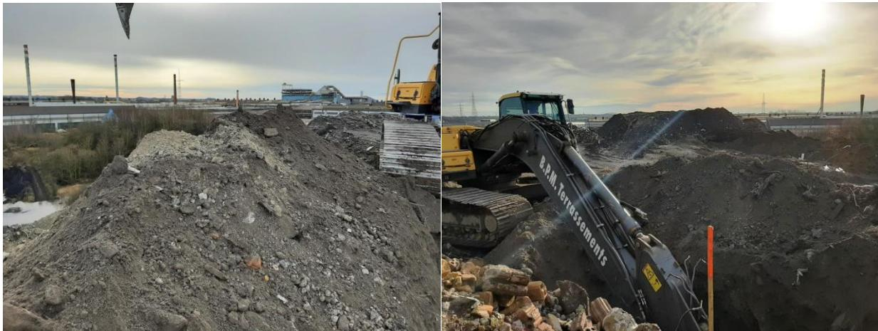
Photograph 1: sampling up to 5m using excavator (B.P.M. Terrassements)
