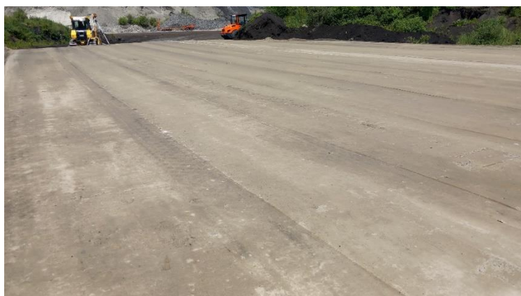
Figure 8: The two first test slabs before the final testing
