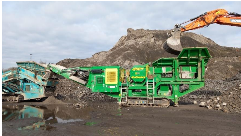
Figure 7: Jaw crusher before screening
